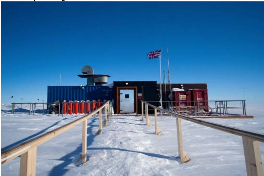
Photo 2: Halley V and the Laws Platform which housed the living accommodation, kitchen, gym, library, workshops and dining area. Halley V was actually built on steel legs, which were jacked each year to keep the platform above snow level. However with Halley VI being built to replace Halley V the decision was made not to jack the building and so for 3 years the snow slowly built up around the base
